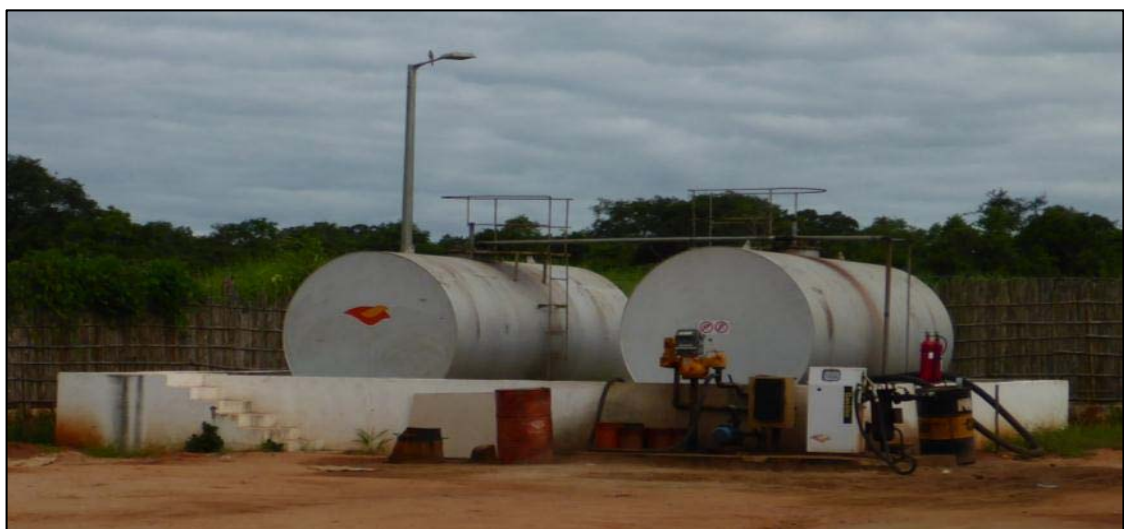
Figure 8-5: Existing Fuel Storage
