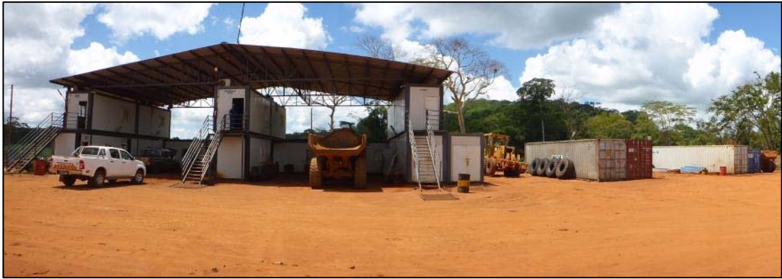
Figure 8-3: Existing Maintenance Workshop
