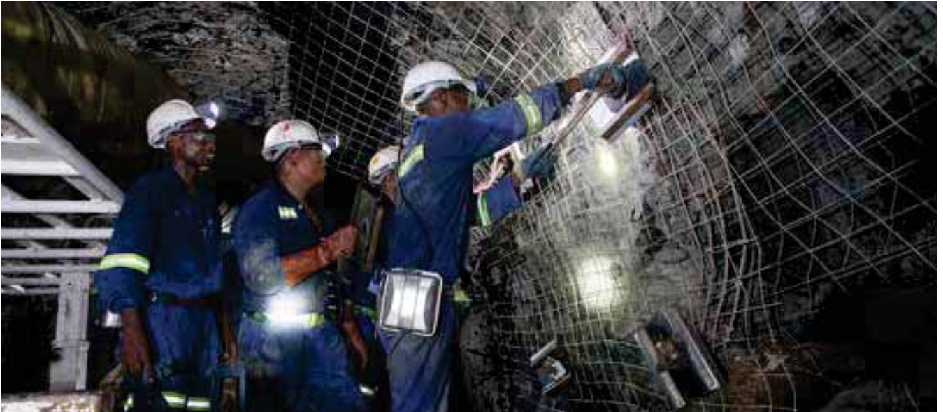
Lining the kimberlite tunnels with safety meshing.
