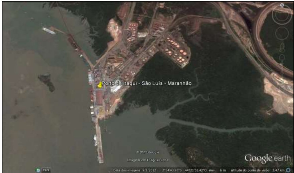
Figure 18.6 Satellite image of the port at Itaquí
