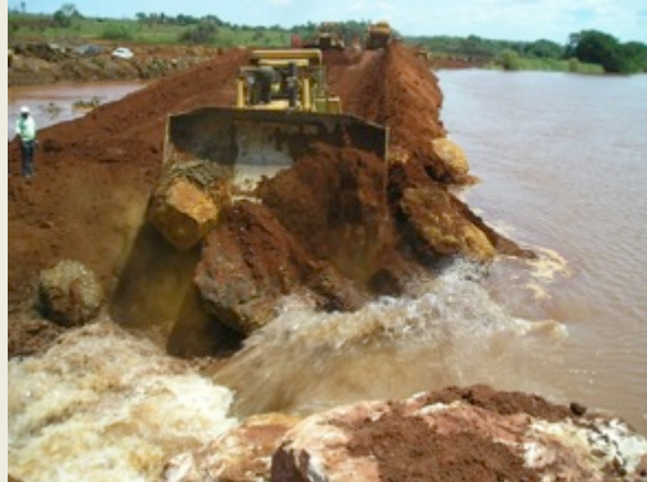
Figure 78 - Luembe River diversion: closing the dyke - Chimbongo project, October 2008 (Fernando Vieira photo).
