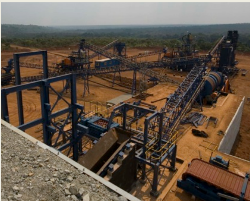
Figure 19 - Installation of the tuff plant in the Camatchia mine.
