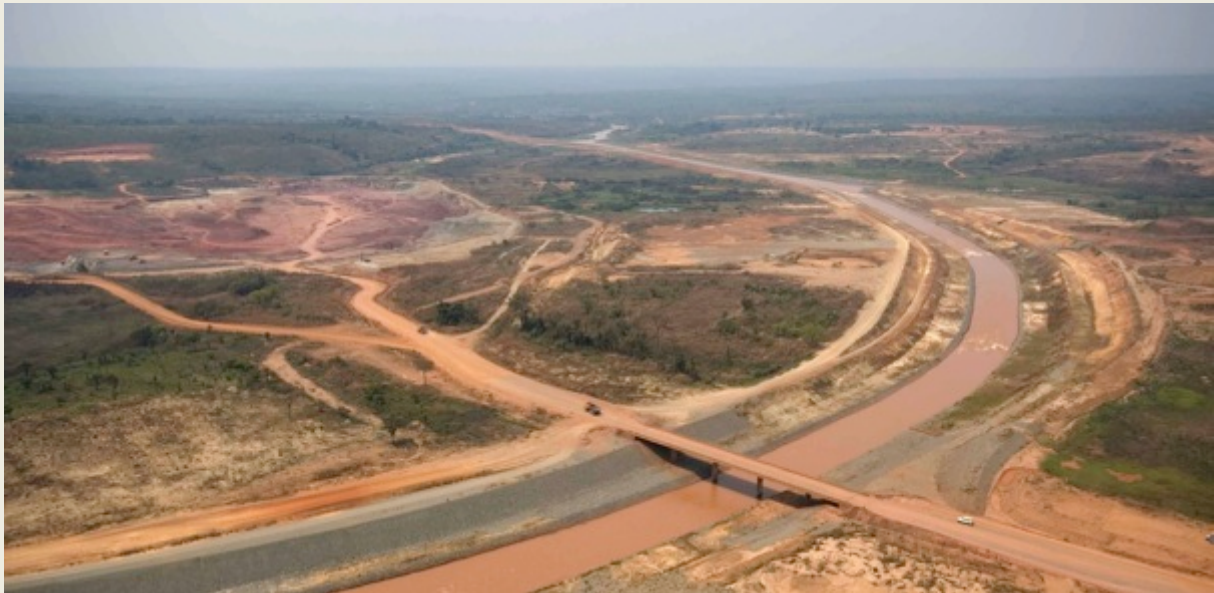
Figure 20 - The Camatchia kimberlite mine in September 2008: Chicapa River diversion channel and bridge in foreground and the pit in left background.
